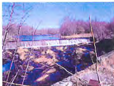
Sawmill Dam before construction
